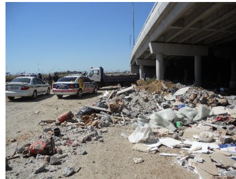
Figure 15 The M5 Birdge area was full of dumping
