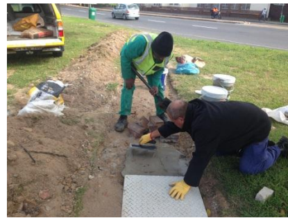
Figure 22 New pathways are constructed
