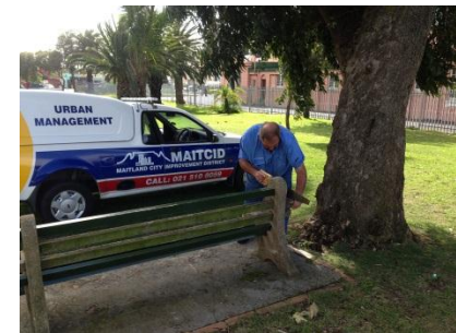
Figure 24 Repairing infrastructure in Maitland Park
