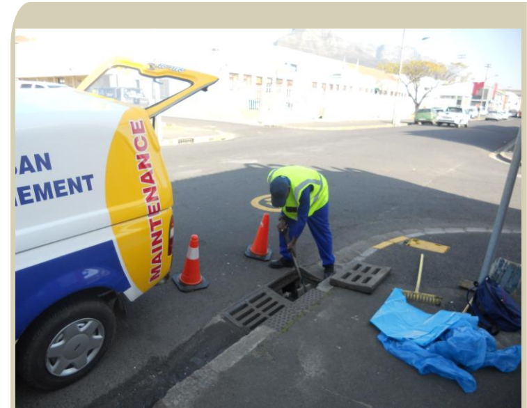
Figure 34 The urban environment needs constant monitoring and management. Miatcid will continue to work with the City of Cape Town to manage the area and address defects for rehabilitation.
