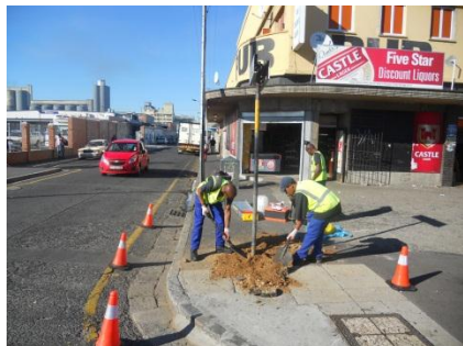
Figure 21 Maitland CID repairs public infrastructure
