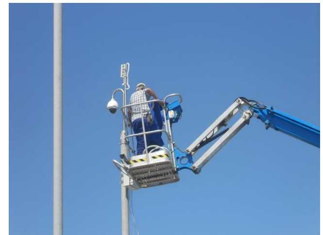
Figure 43 Maitcid CCTV cameras being installed
